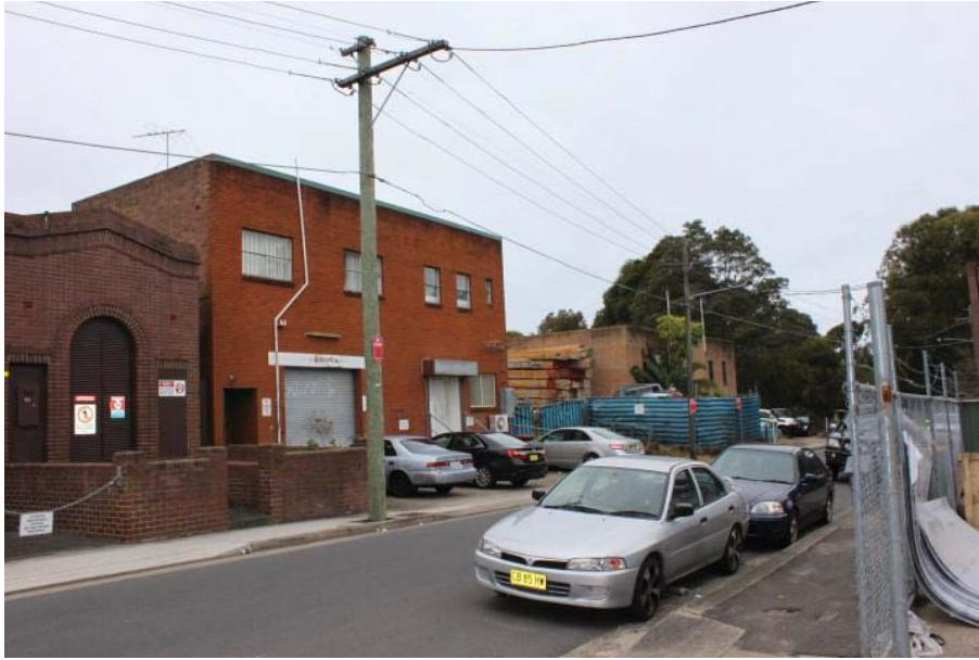
Figure 3: The subject Site from Close Street
