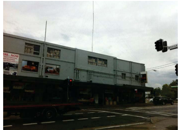
Ausland Furniture of the western front part of the site
